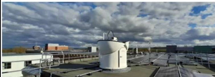
TCCON dome installed on RAL roof
